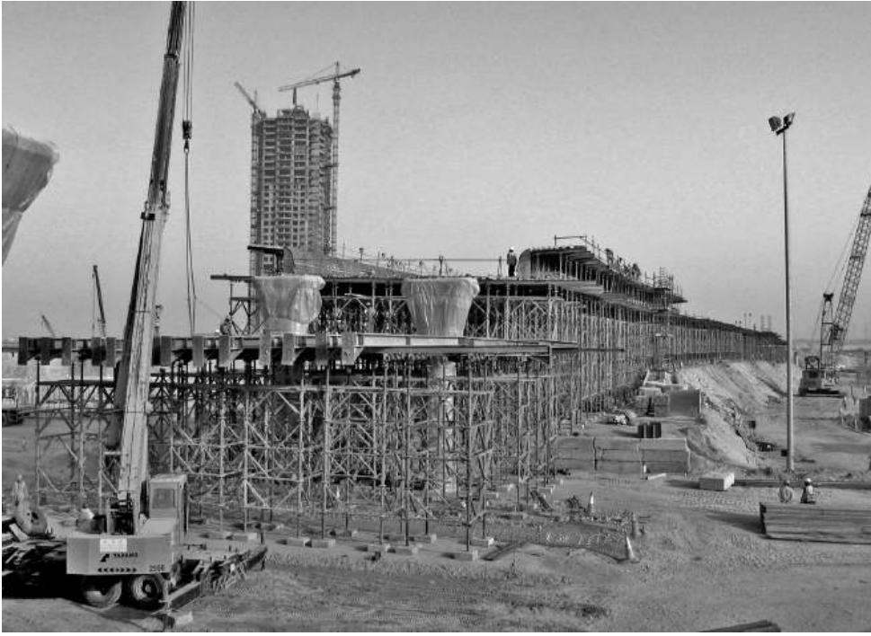
Figure 11.5 Formwork being installed
