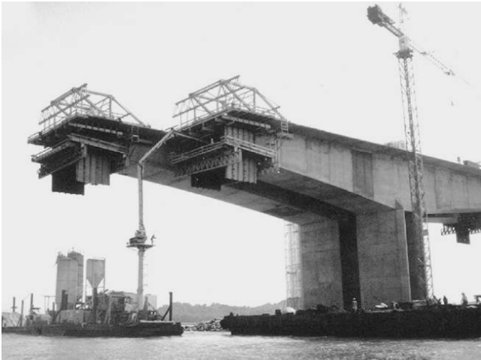
Figure 7.3 In situ box girder
