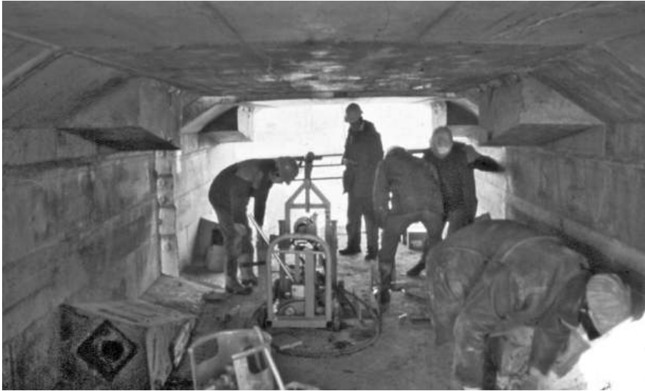
Figure 13.31 View inside box girder as segment is being positioned
