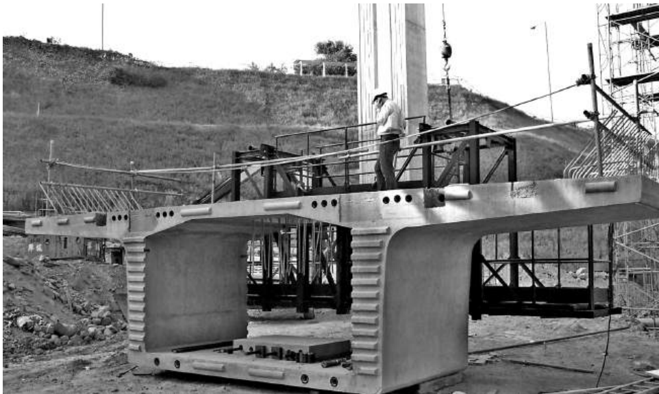
Figure 13.57 Stressing platform on segment
