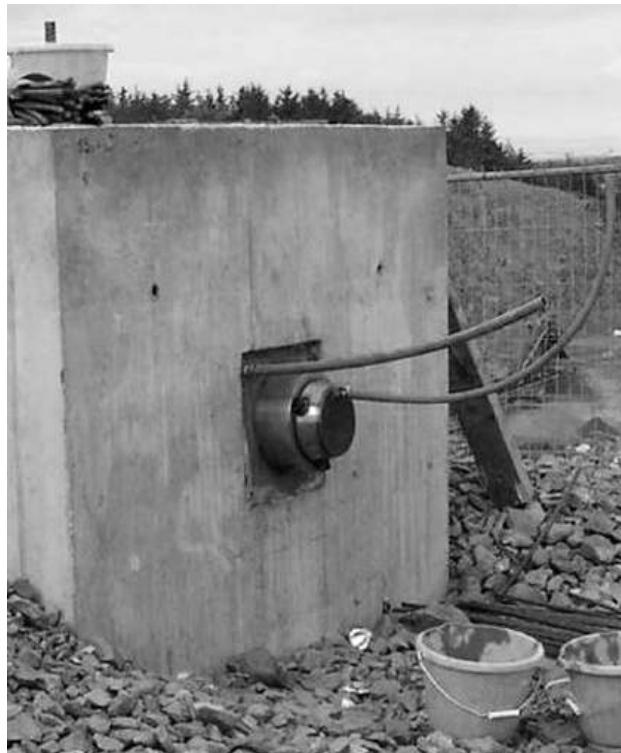
Figure 4.6 Anchor cap with grout inlet
