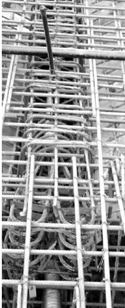
Figure 6.5 Dead-end anchorage reinforcement
