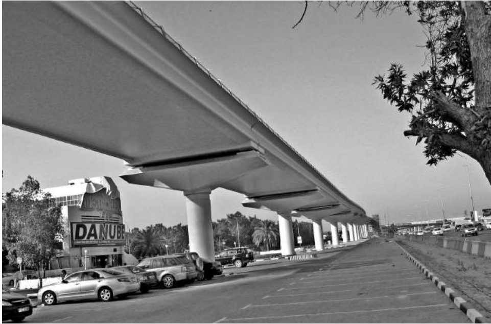
Figure 13.5 Dubai LRT U-trough deck
