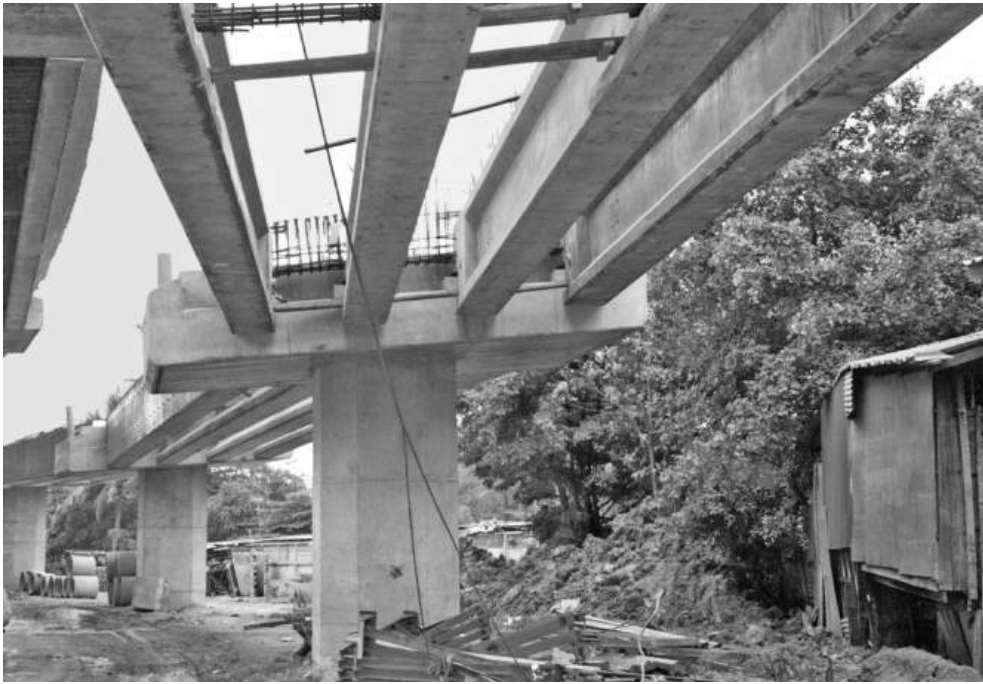
Figure 10.11 Precast beams on crosshead prior to casting diaphragms and deck slab
