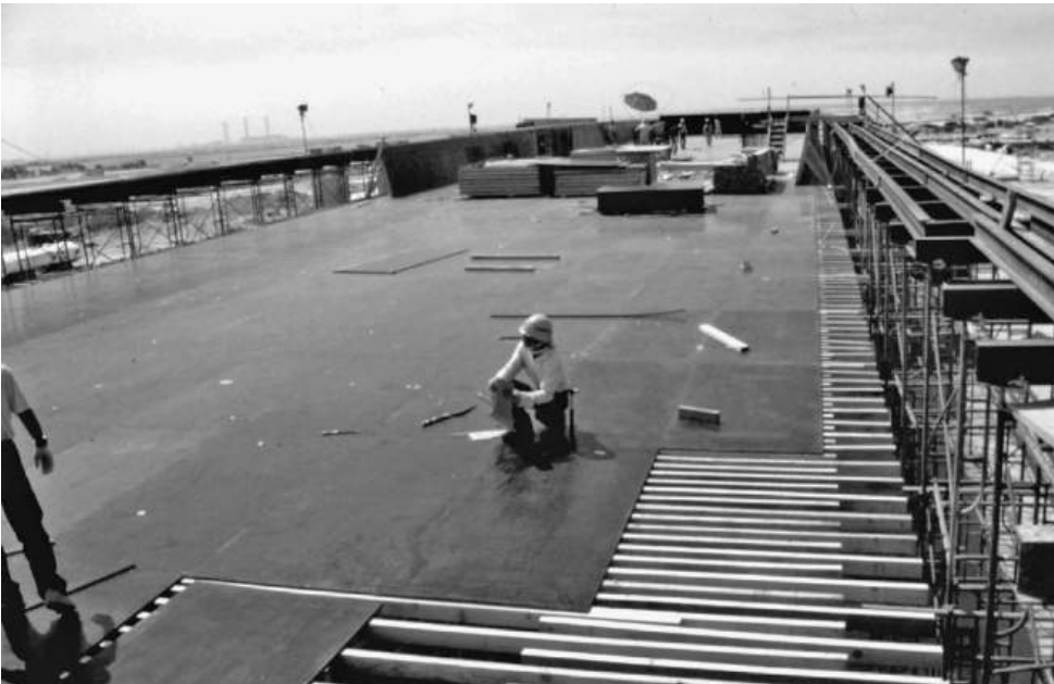
Figure 11.5 Formwork being installed
