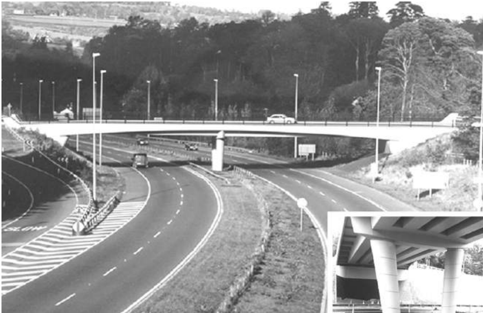
Figure 1.4 Killarney Overbridge, Ireland (reproduced courtesy of Roughan & O'Donovan, Dublin, copyright reserved)
