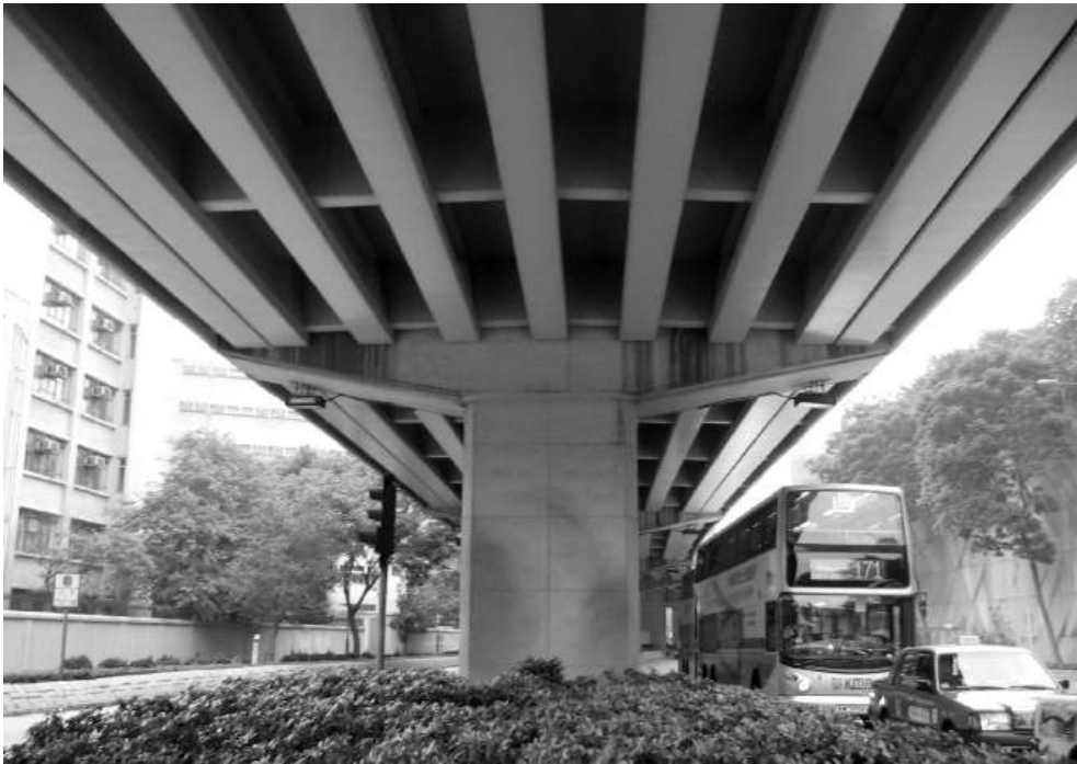
Figure 10.1 Typical precast beam deck
