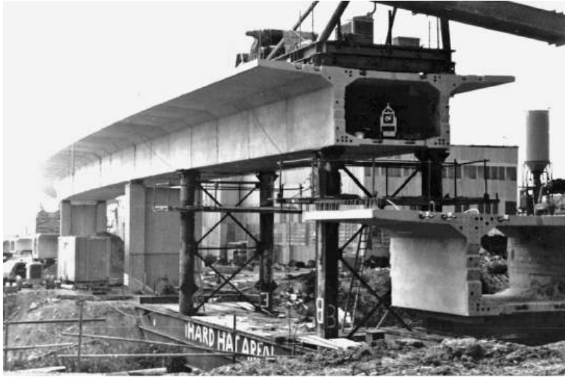
Figure 13.49 Progressive placing of segments with props
