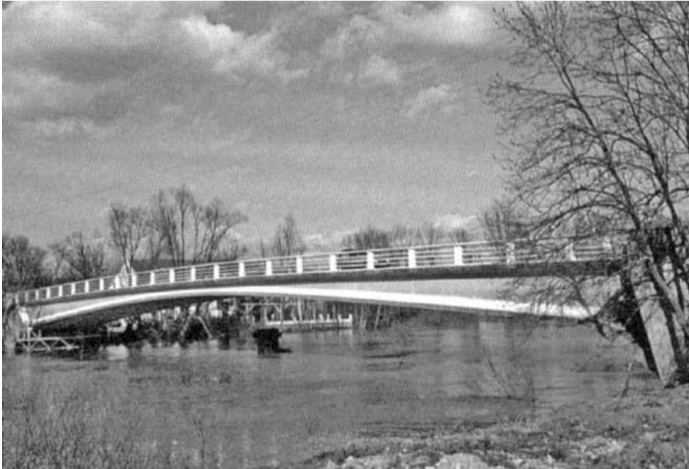
Figure 1.12 Annet Bridge, France (reproduced courtesy of Freyssinet International, copyright reserved)
