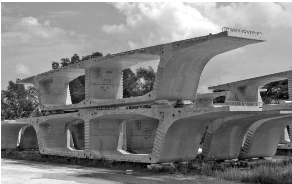
Figure 13.19 Segments in storage yard
