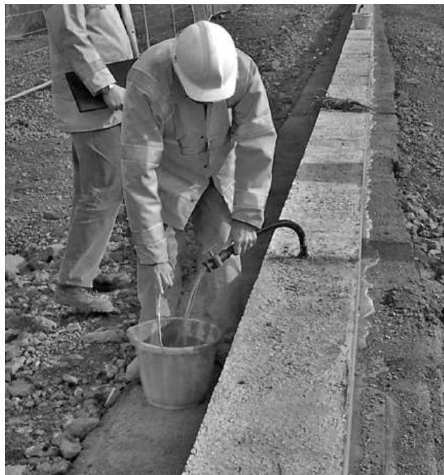
Figure 4.9 Grout being collected at an intermediate vent point
