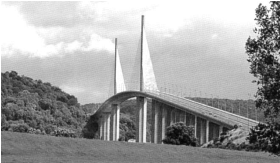
Figure 1.18 Brotonne Bridge, France (reproduced courtesy of Freyssinet International, copyright reserved)
