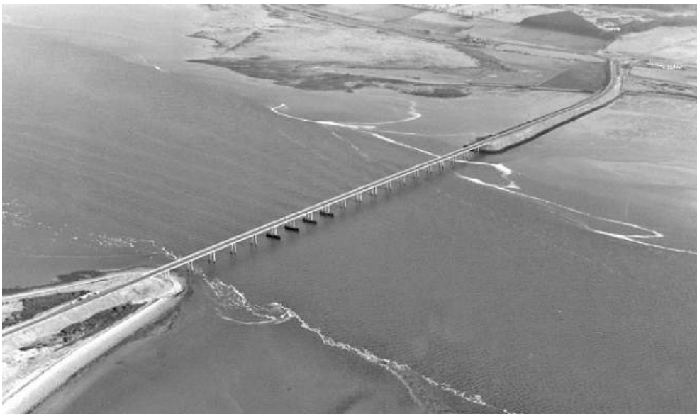
Figure 1.17 Dornoch Firth crossing, Scotland (reproduced courtesy of Tony Gee and Partners LLP, copyright reserved)
