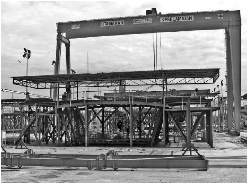
Figure 13.14 Reinforcement assembly jig
