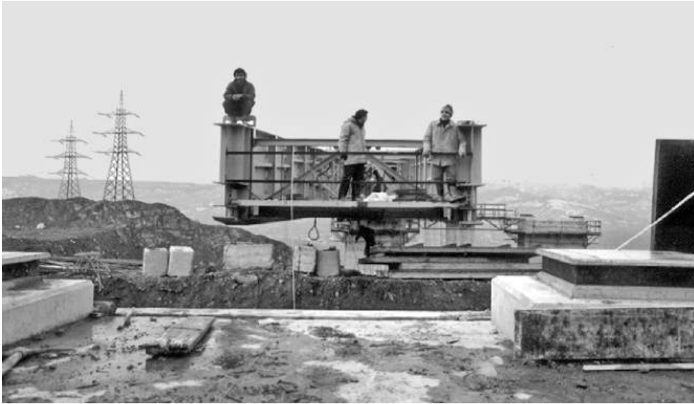
Figure 15.13 Temporary bearings for launch
