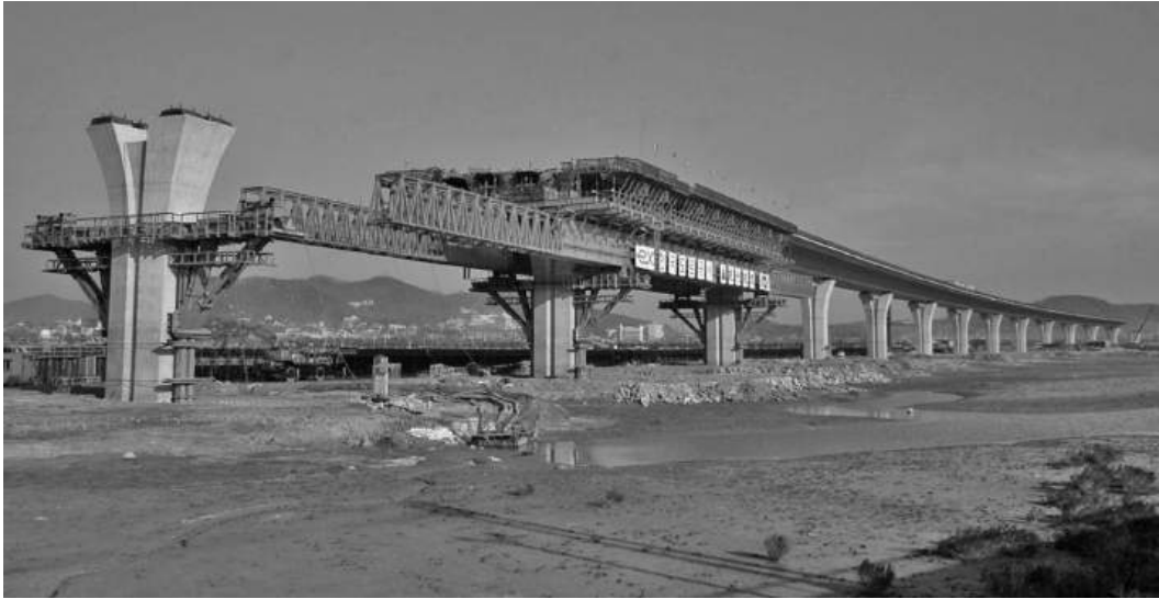
Figure 12.7 Gantry support for formwork (reproduced courtesy of C.S. Park, copyright reserved)
