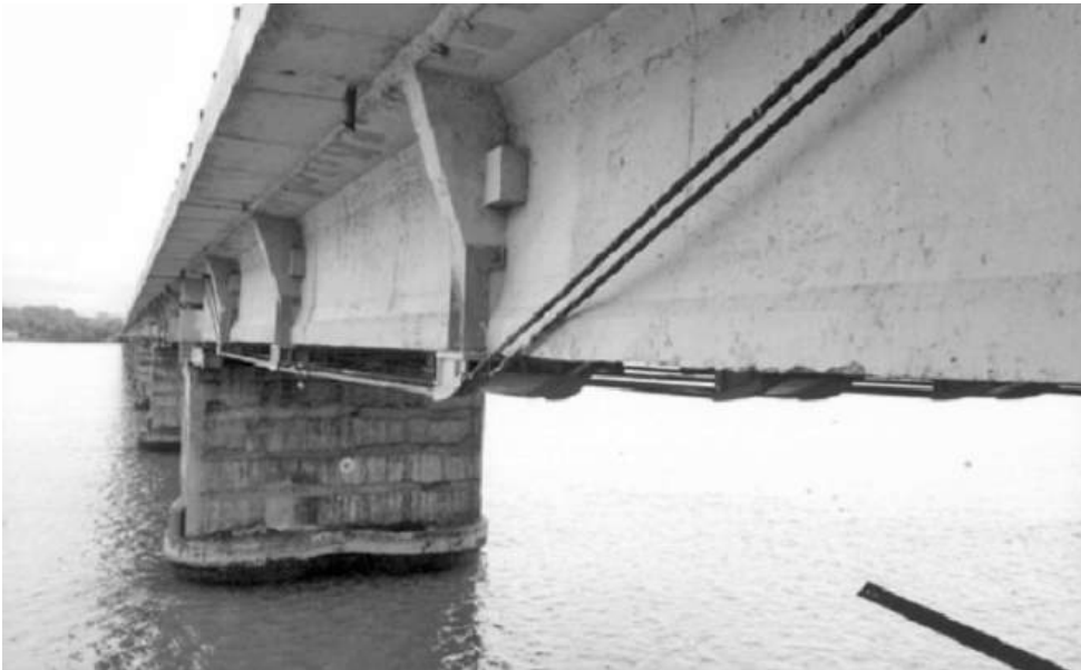
Figure 6.20 Steel deviator (reproduced courtesy of Hyder Consulting (UK) Ltd, copyright reserved)
