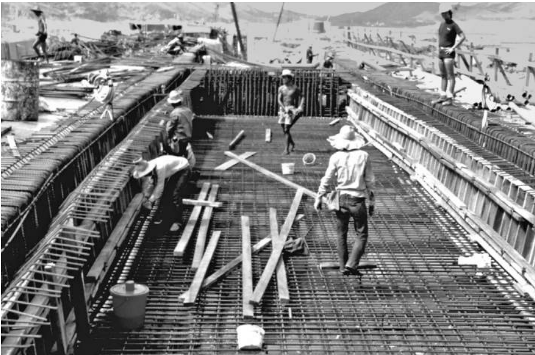
Figure 12.8 Reinforcement and ducts being placed
