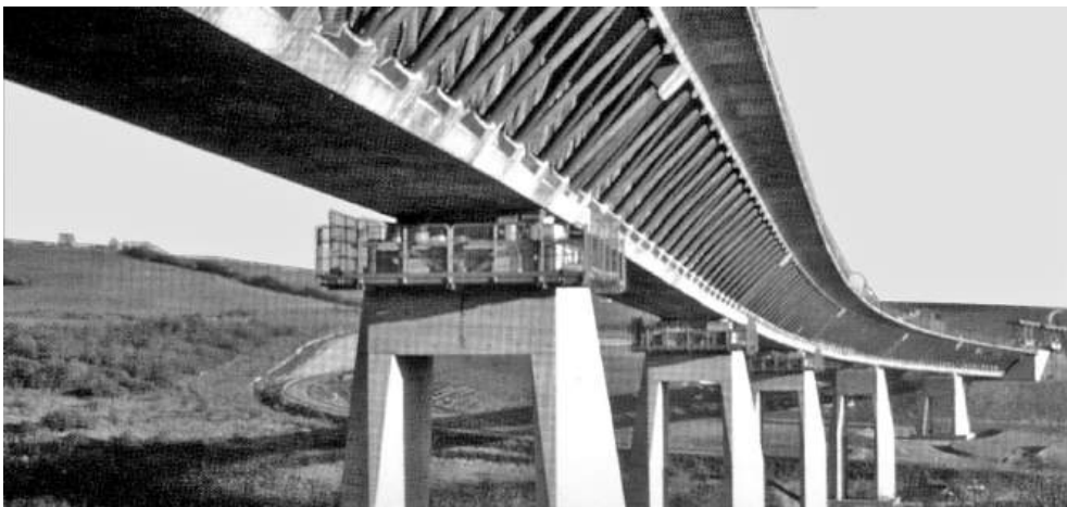
Figure 17.6 Brouha Bridge, France (reproduced courtesy of VSL International, copyright reserved)
