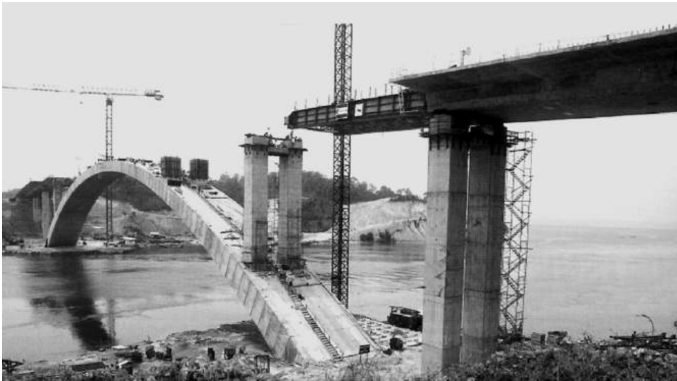
Figure 17.9 Barelang Bridge, Indonesia (reproduced courtesy of Freyssinet International, copyright reserved)
