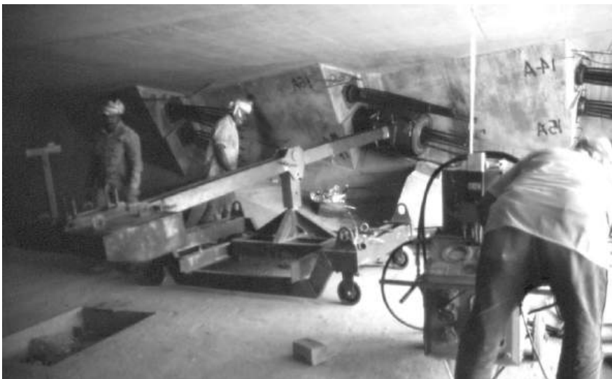
Figure 2.15 Placing of large prestressing jack onto tendon
