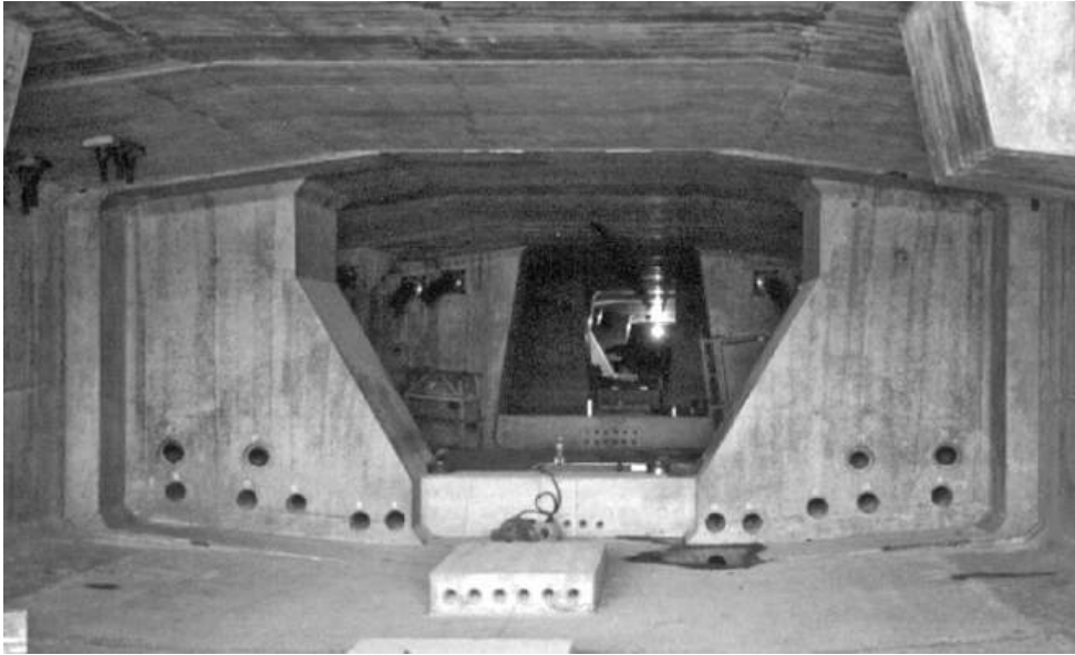
Figure 3.8 Access through box girder diaphragms
