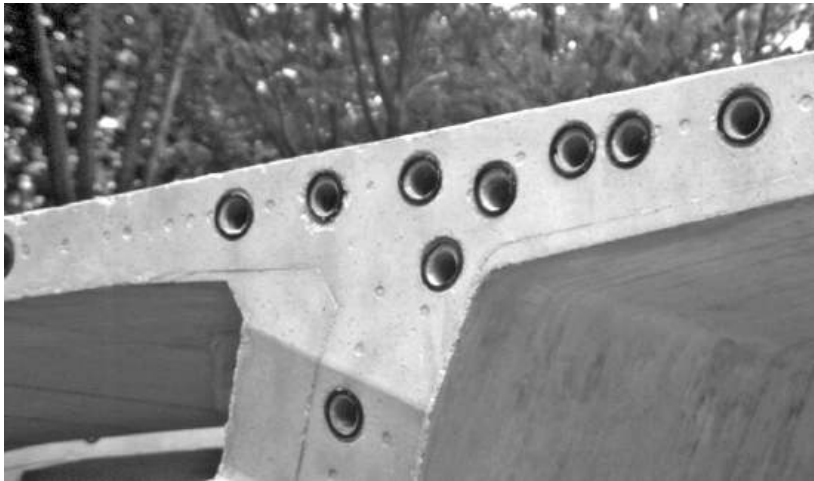
Figure 13.28 'O' rings around ducts at segment joints
