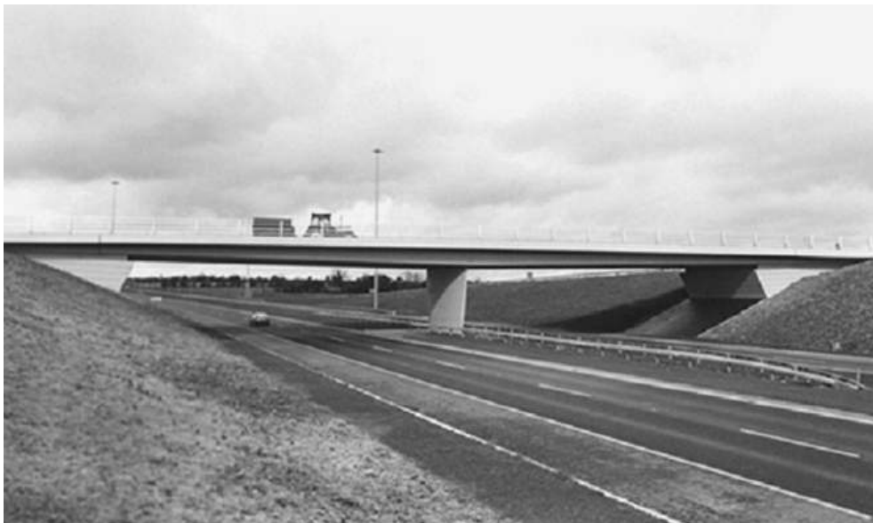
Figure 9.1 Balbriggan Bridge, Ireland (reproduced courtesy of Roughan & O'Donovan, Dublin, copyright reserved)
