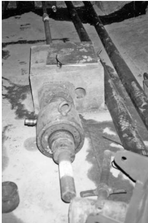
Figure 2.15 Placing of large prestressing jack onto tendon
