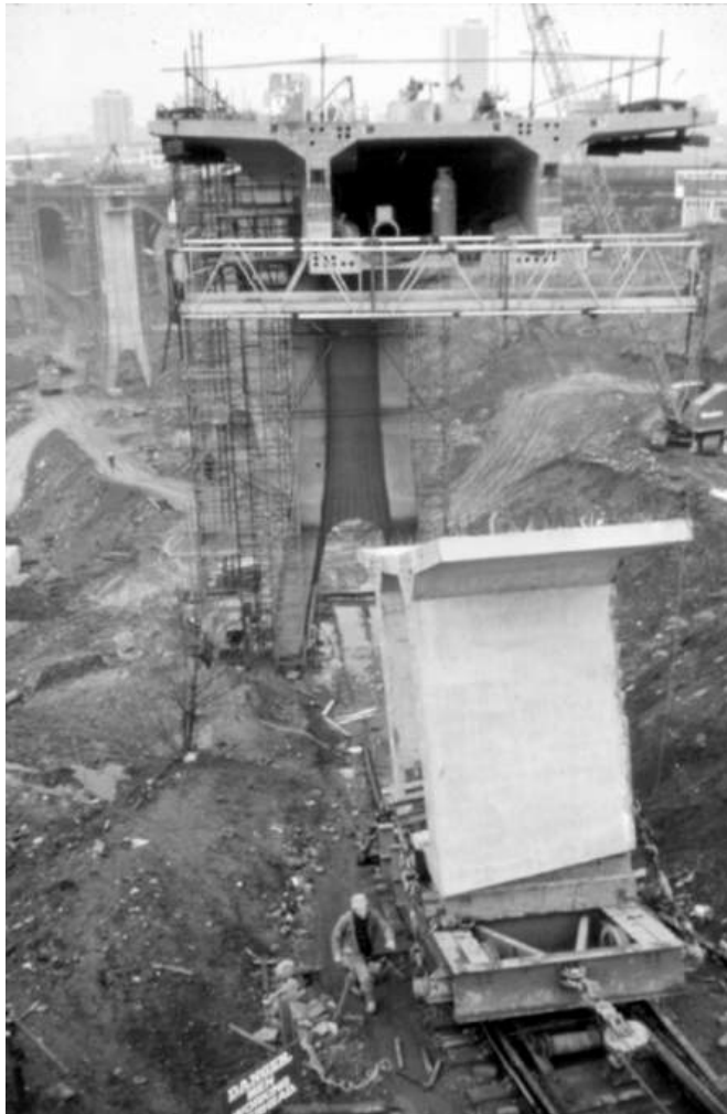
Figure 13.24 Segment positioned on rail mounted bogey
