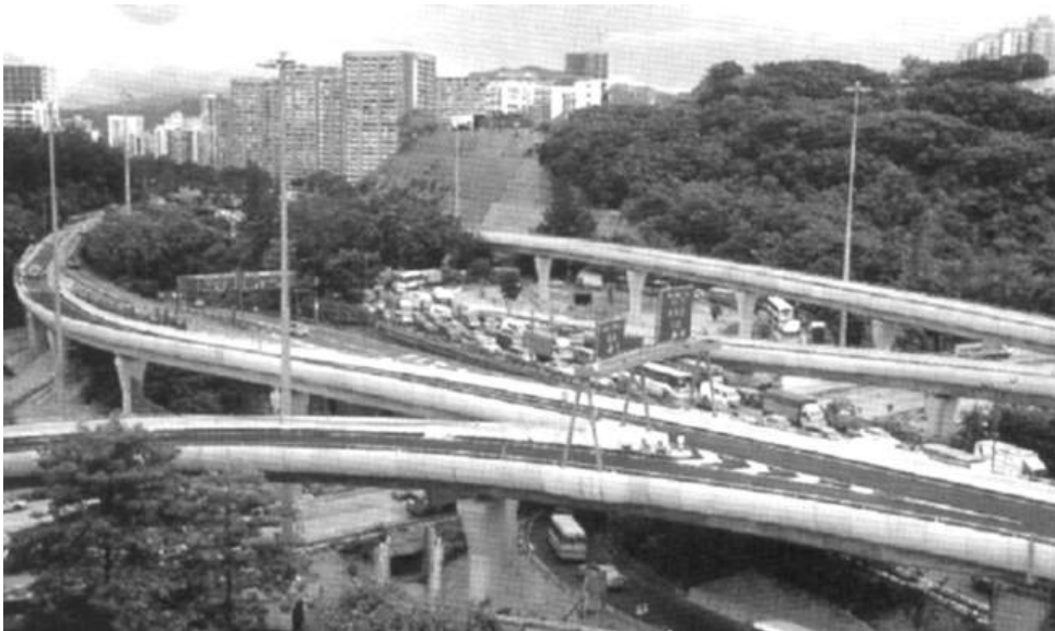
Figure 13.4 Hung Hom Bypass and Princess Margaret Road Links, Hong Kong (reproduced courtesy of Hyder Consulting (UK) Ltd, copyright reserved)
