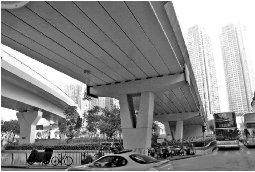
Figure 1.16 Precast beam flyover in Hong Kong
