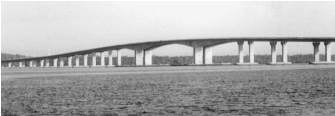
Figure 12.2 Malaysia–Singapore Second Crossing (reproduced courtesy of Hyder Consulting (UK) Ltd, copyright reserved)
