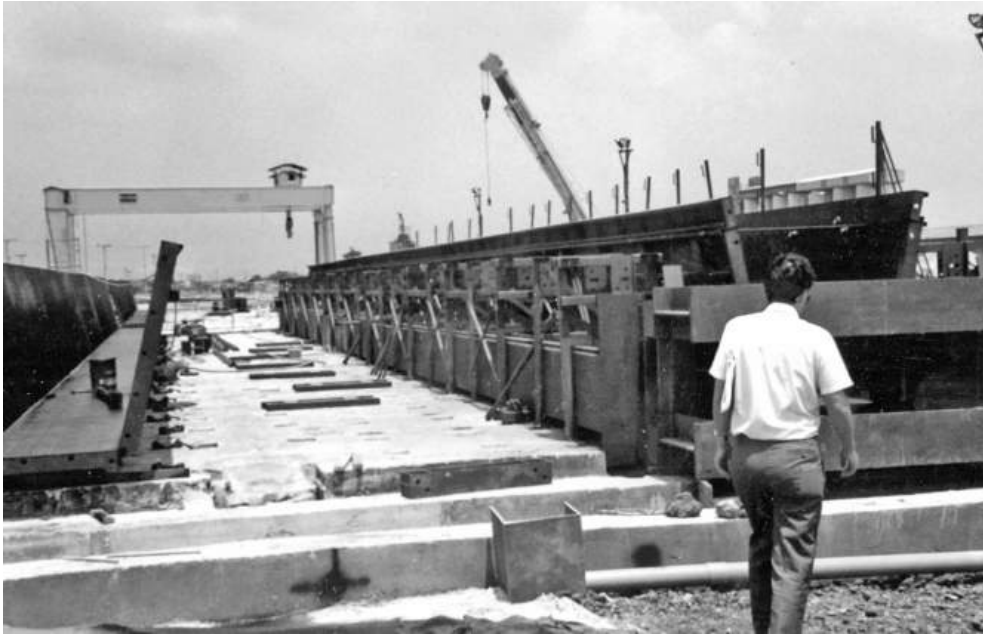
Figure 10.16 Shutter with strands anchored at ends
