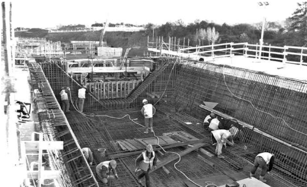
Figure 15.11 Casting cell looking towards deck
