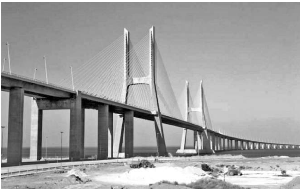
Figure 16.2 Vasco da Gama Bridge, Portugal (reproduced courtesy of Yee Associates, copyright reserved)
