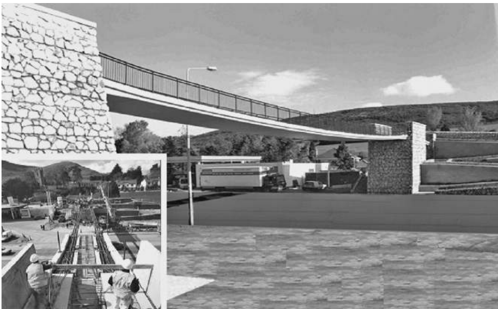
Figure 17.12 Stressed ribbon footbridge, Ireland (reproduced courtesy of Roughan & O'Donovan, Dublin, copyright reserved)
