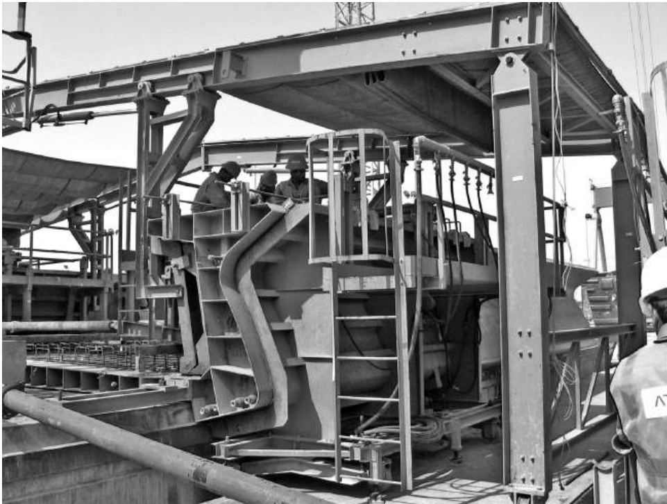
Figure 13.13 Long line formwork
