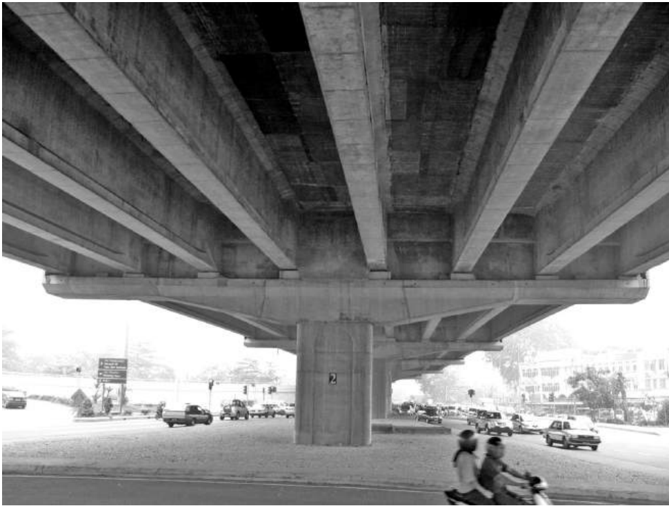
Figure 6.15 'U' beam diaphragm
