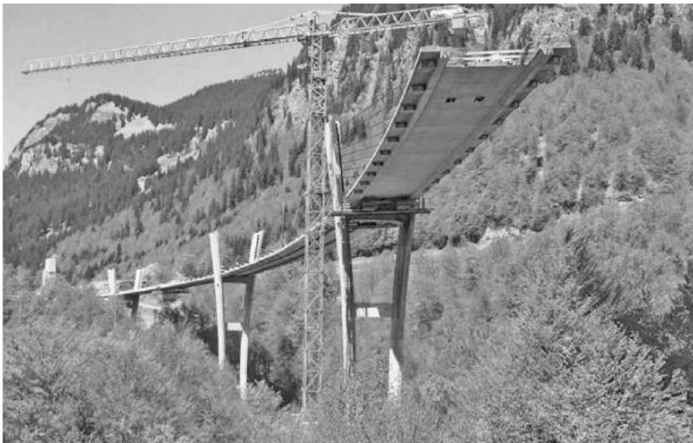
Figure 17.3 Sunniberg Bridge, Switzerland (reproduced courtesy of BBR Systems Ltd, copyright reserved)
