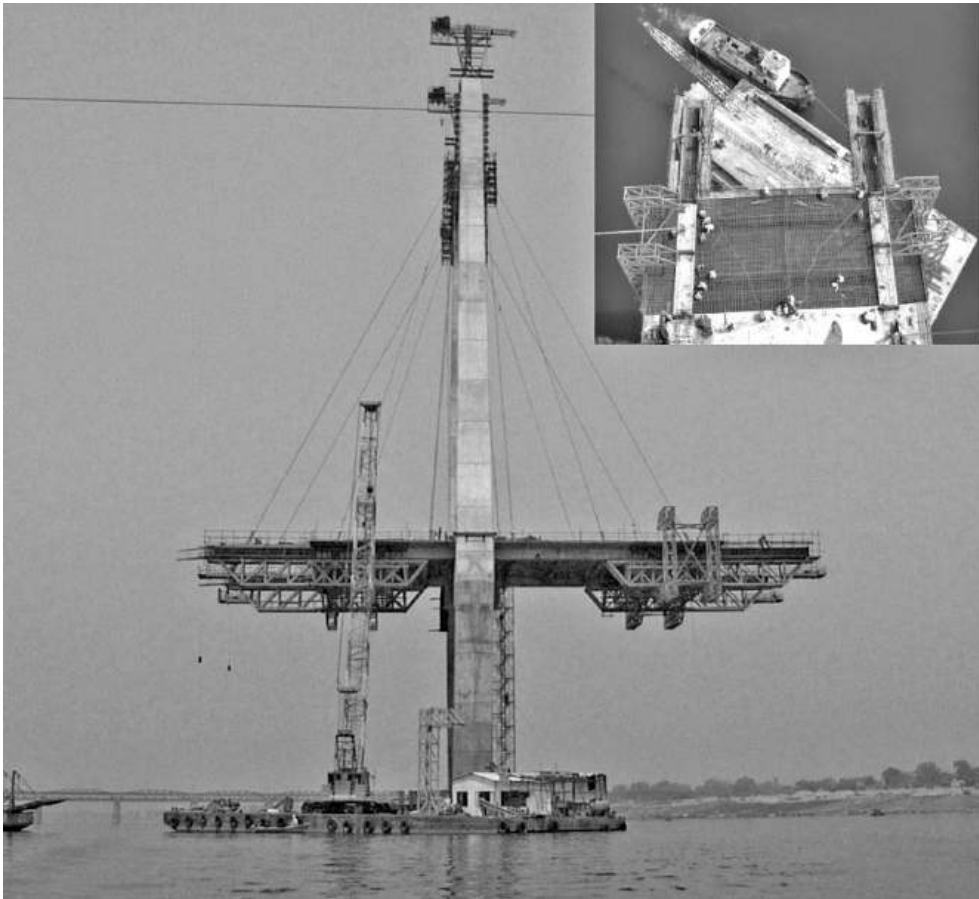
Figure 16.13 Beam-and-slab deck under construction
