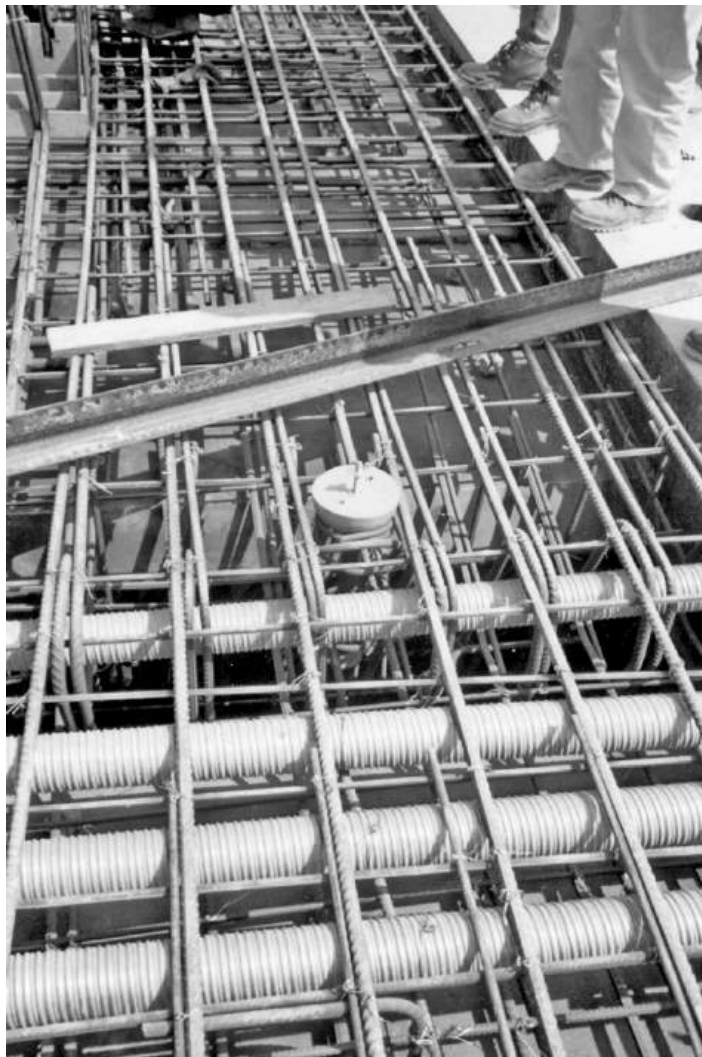
Figure 2.7 Steel ducts inside reinforcement cage
