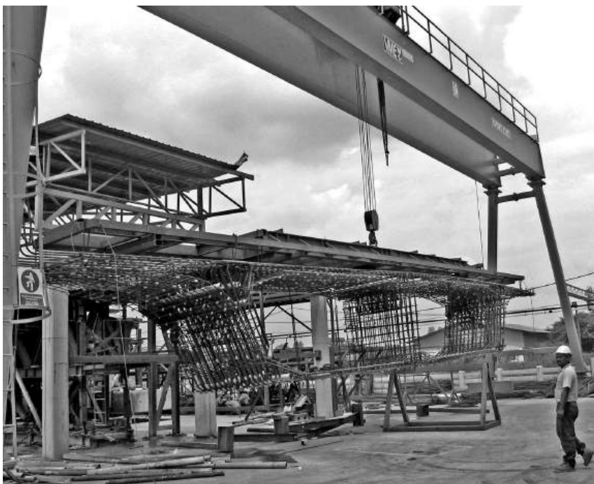
Figure 13.15 Reinforcement cage being lifted and moved to casting cell
