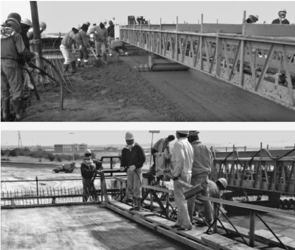
Figure 11.9 Deck finishing machine
