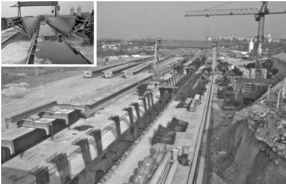
Figure 10.14 Casting bed for pre-tensioned beams
