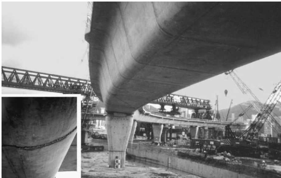
Figure 13.32 Close up of joint after segment erected
