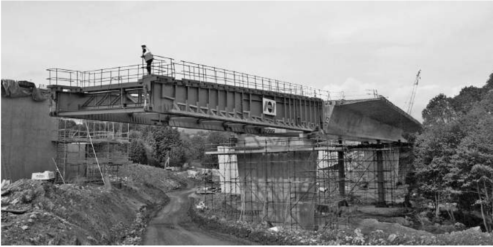
Figure 7.5 Incrementally launched box girder
