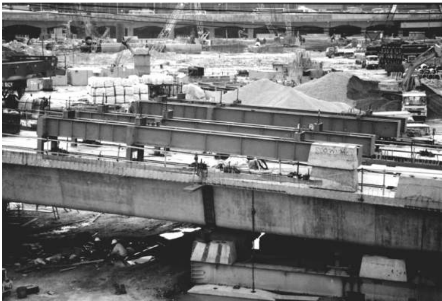
Figure 13.44 Frame to align cantilevers
