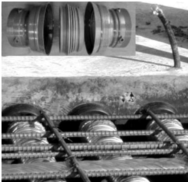
Figure 13.29 Liaseal Coupler (reproduced courtesy of Freyssinet International, copyright reserved)
