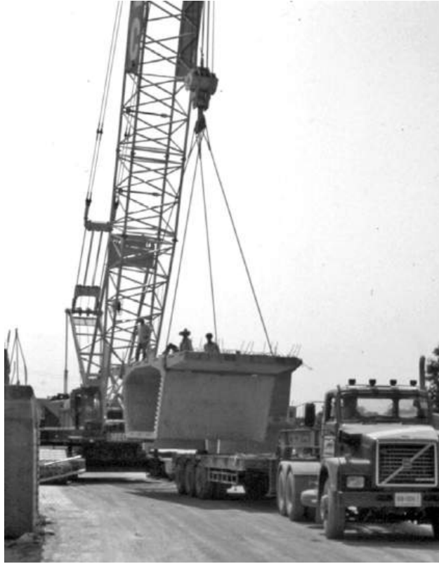
Figure 13.22 Segments lifted by crane at storage yard
