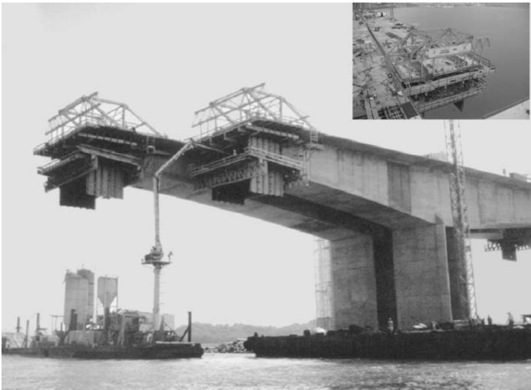
Figure 12.14 Travelling form on deck
