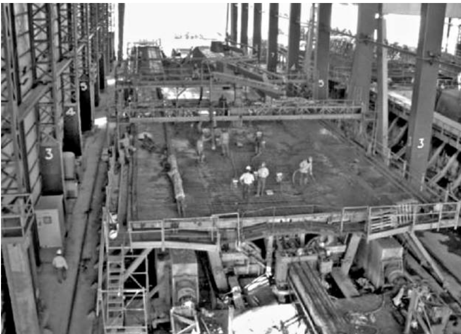
Figure 14.7 Unit being concreted (reproduced courtesy of VSL Intrafor Asia, copyright reserved)
