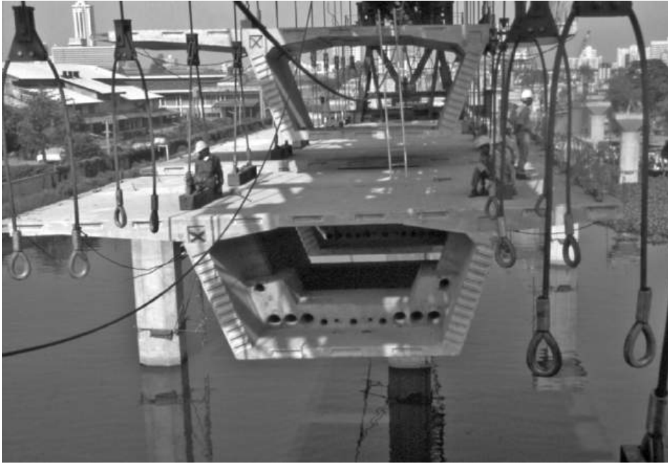
Figure 13.46 Segments hang from gantry
