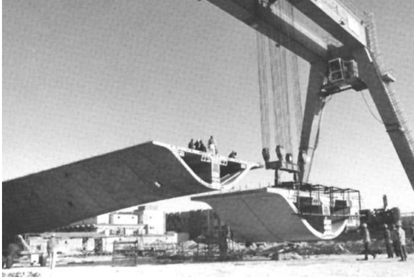
Figure 13.40 Precast segments erected by lifting frame
