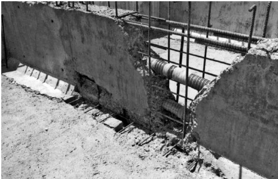
Figure 18.7 Honeycombing and voids in concrete
