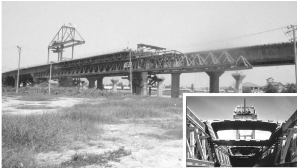
Figure 13.47 Underslung truss for span-by-span erection
