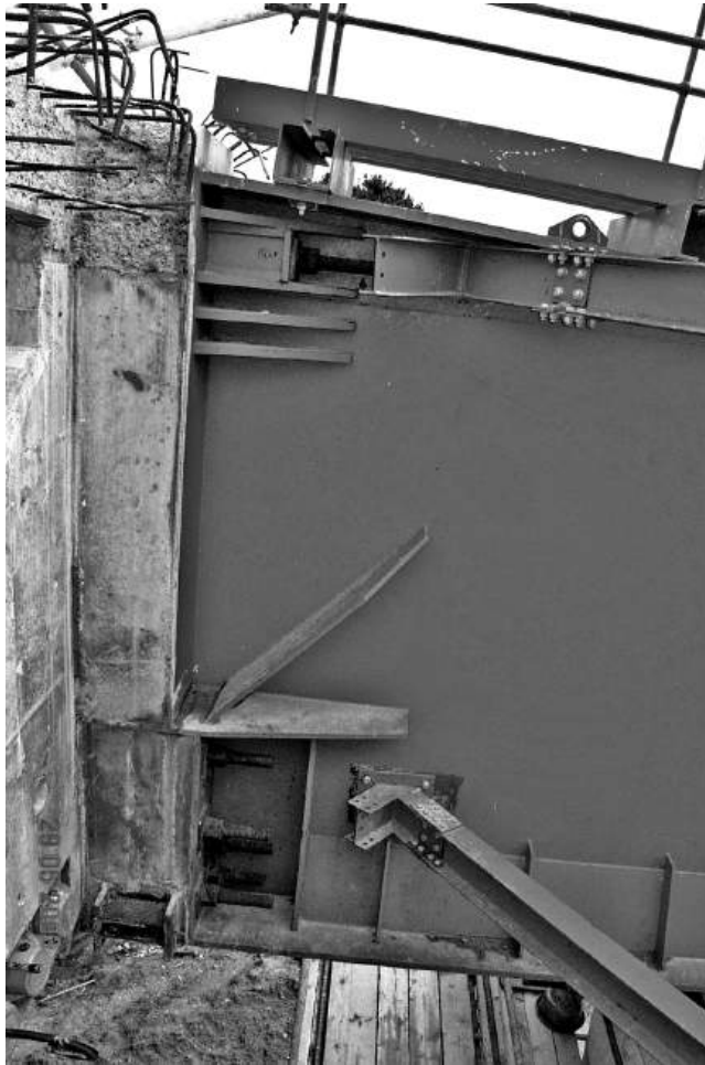
Figure 15.8 Launch nose connection to the deck
