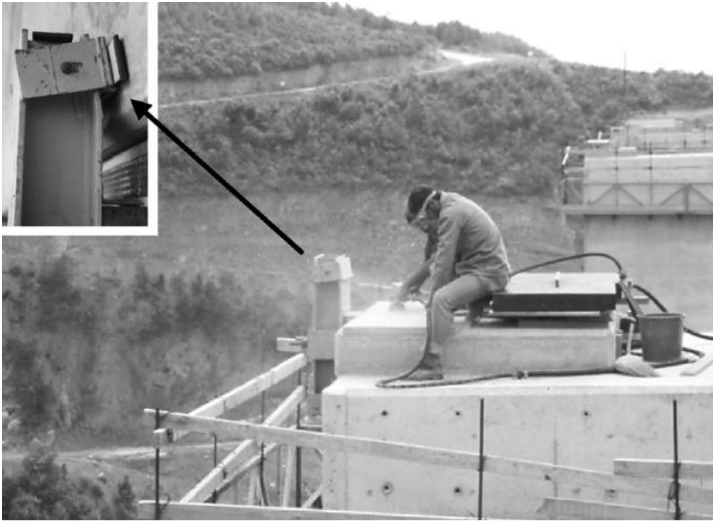
Figure 15.17 Guides fixed to piers and bearing plinths being prepared
