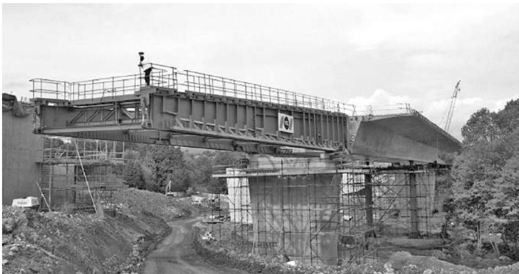
Figure 15.18 Launching nose on deck
