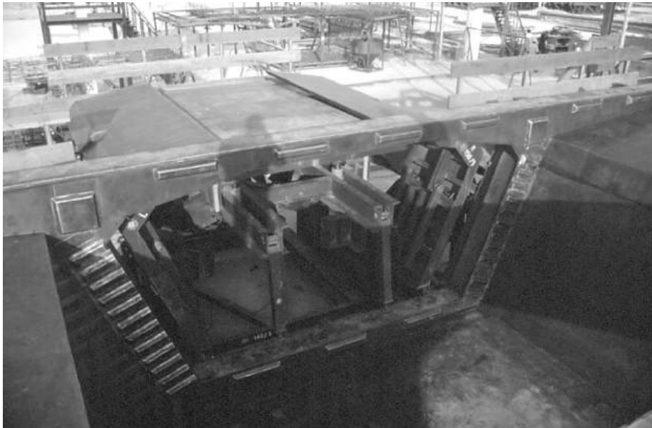
Figure 13.10 Inner shutter ready to slide into position
