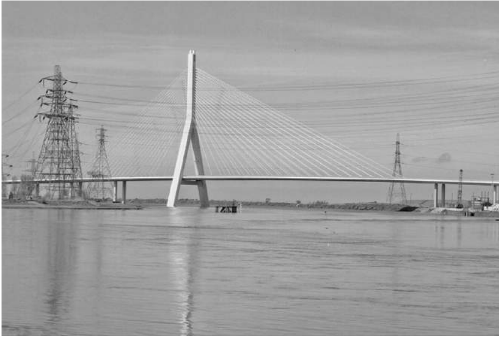
Figure 1.3 River Dee crossing, Wales (reproduced courtesy of Gifford, part of Ramboll, copyright reserved)
