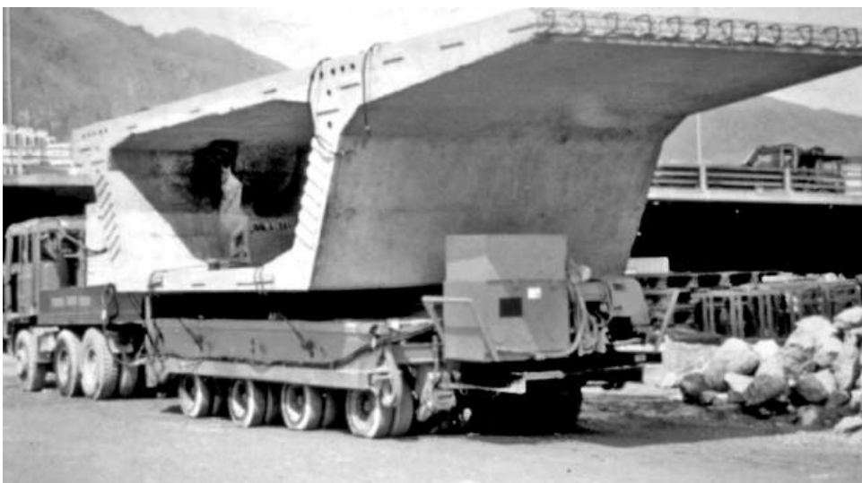
Figure 13.21 Segment on special carrier
