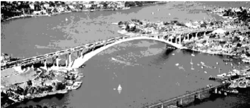
Figure 17.8 Gladesville Bridge, Australia (reproduced courtesy of Maunsell Australia Pty Ltd (a legacy AECOM company), copyright reserved)
