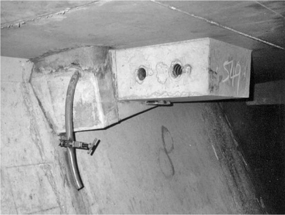
Figure 4.7 Concrete capping to anchorage
