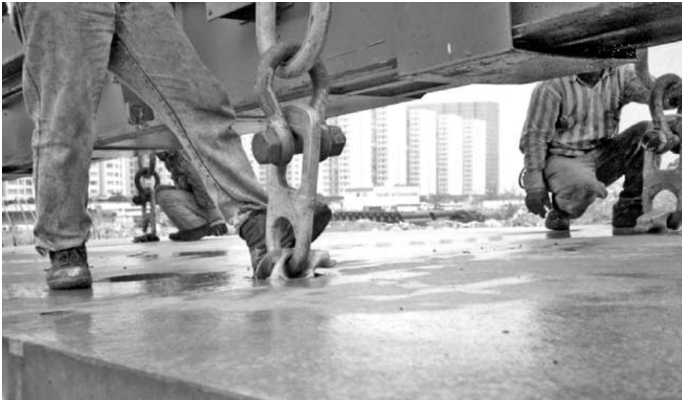
Figure 13.23 Cast-in lifting hooks
