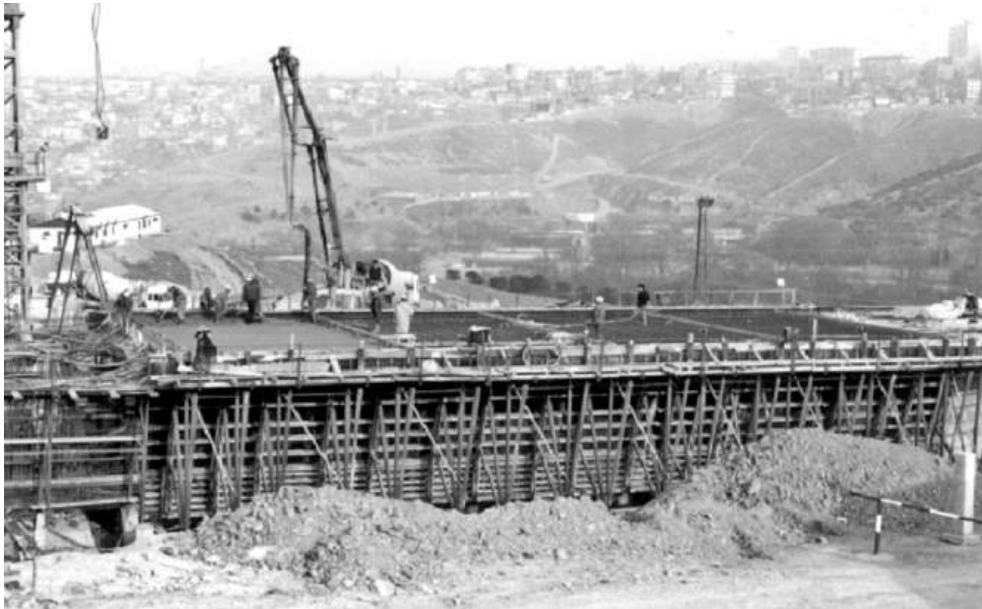
Figure 15.12 Concreting deck slab
