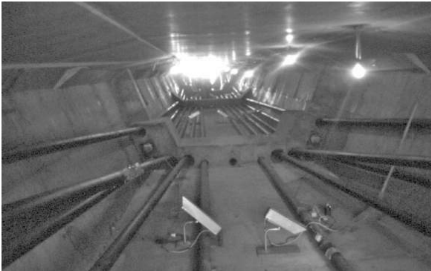
Figure 5.4 External tendons inside box girder
