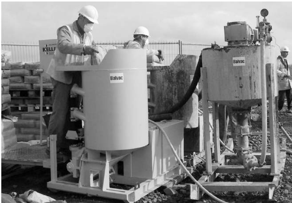
Figure 4.5 Grout-mixing equipment
