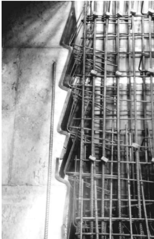
Figure 13.53 Reinforcement for large shear keys
