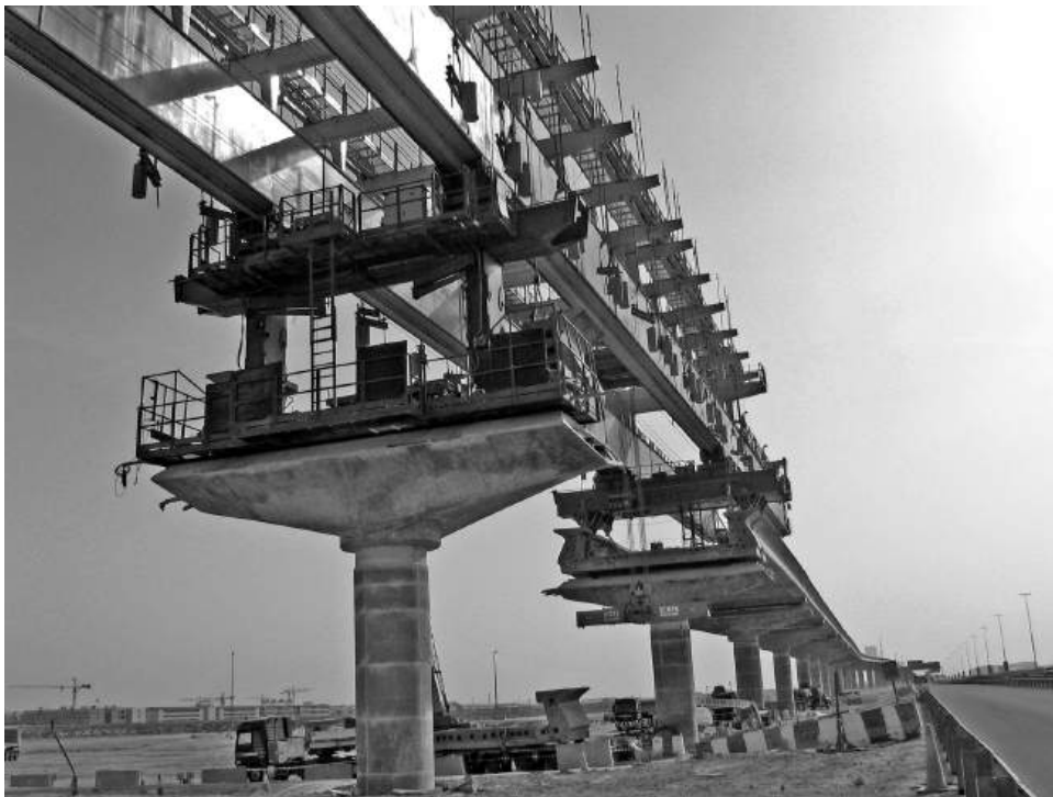
Figure 13.45 Overhead gantry for span-by-span erection
