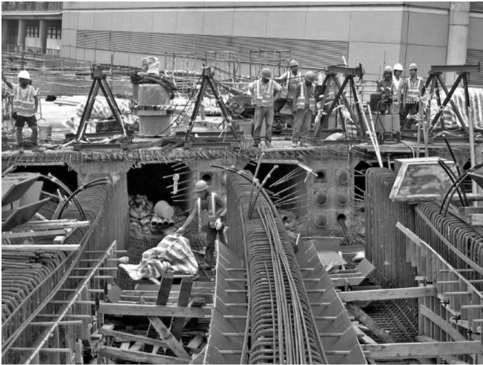
Figure 11.3 Multi-cell box girder bridge
