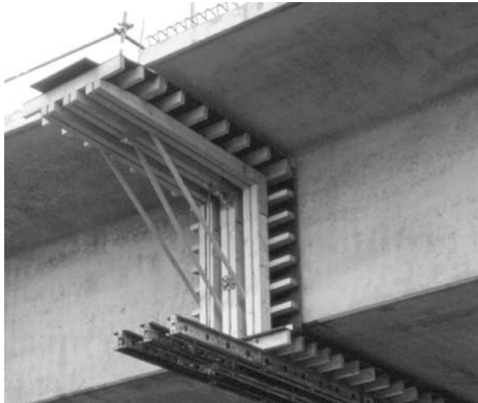
Figure 13.43 Shutter for in situ stitch at midspan
