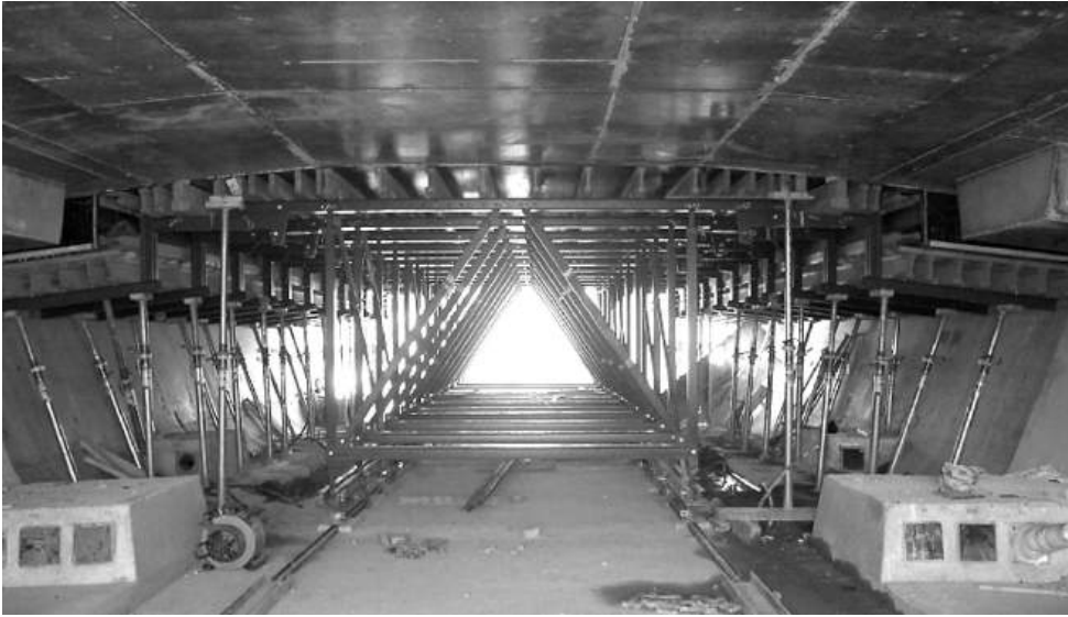
Figure 12.9 Shutter for top slab between webs
