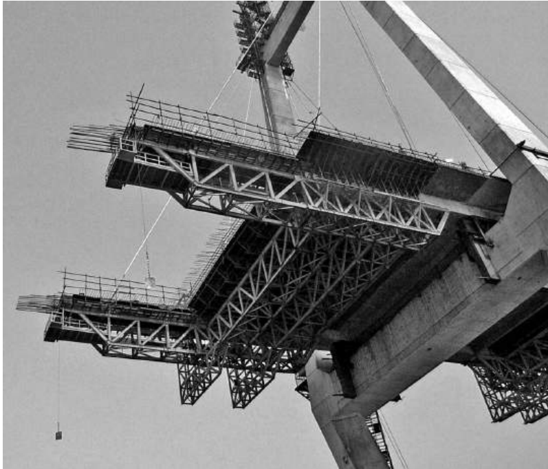
Figure 16.11 Form traveller for casting deck
