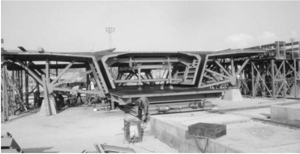
Figure 13.9 Short-line casting bed
