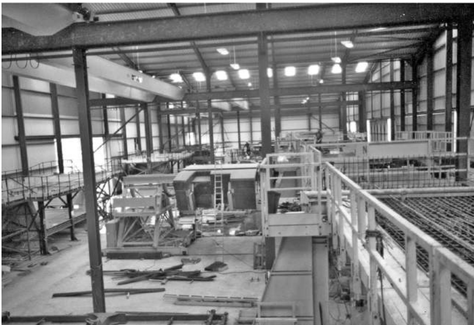
Figure 13.7 General view inside casting yard
