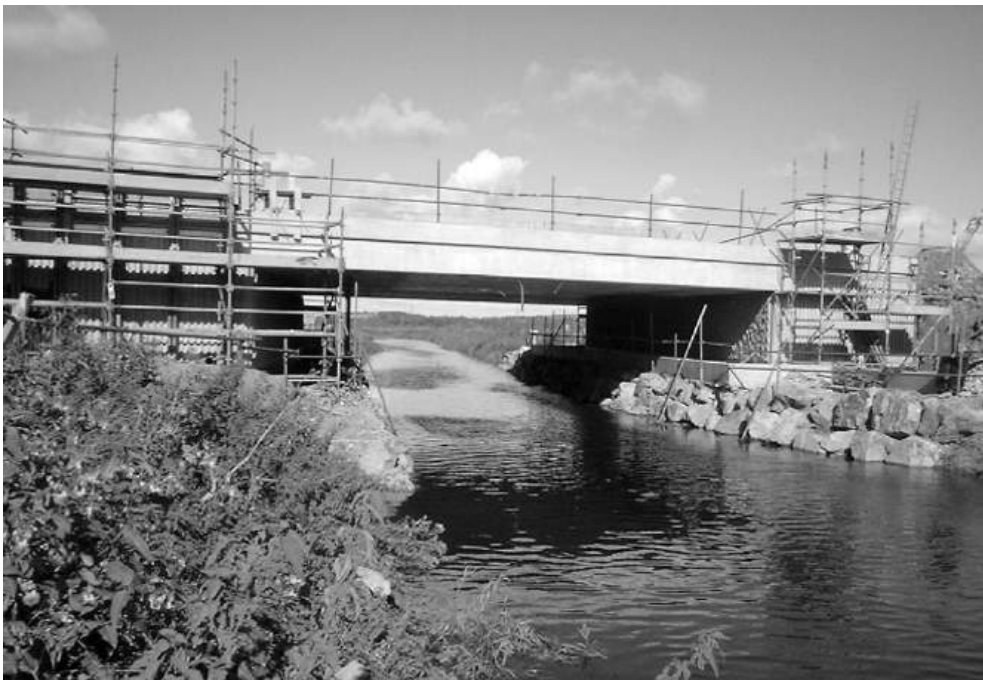
Figure 10.4 Precast beam bridge under construction over river (reproduced courtesy of Hyder Consulting (UK) Ltd, copyright reserved)
