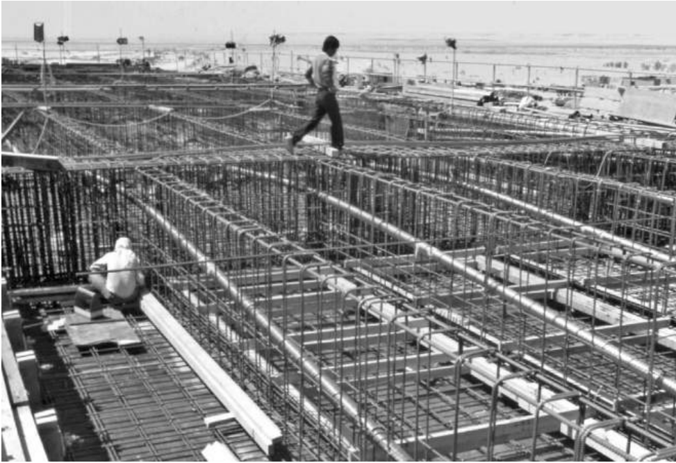
Figure 11.6 Reinforcement and tendon ducts
