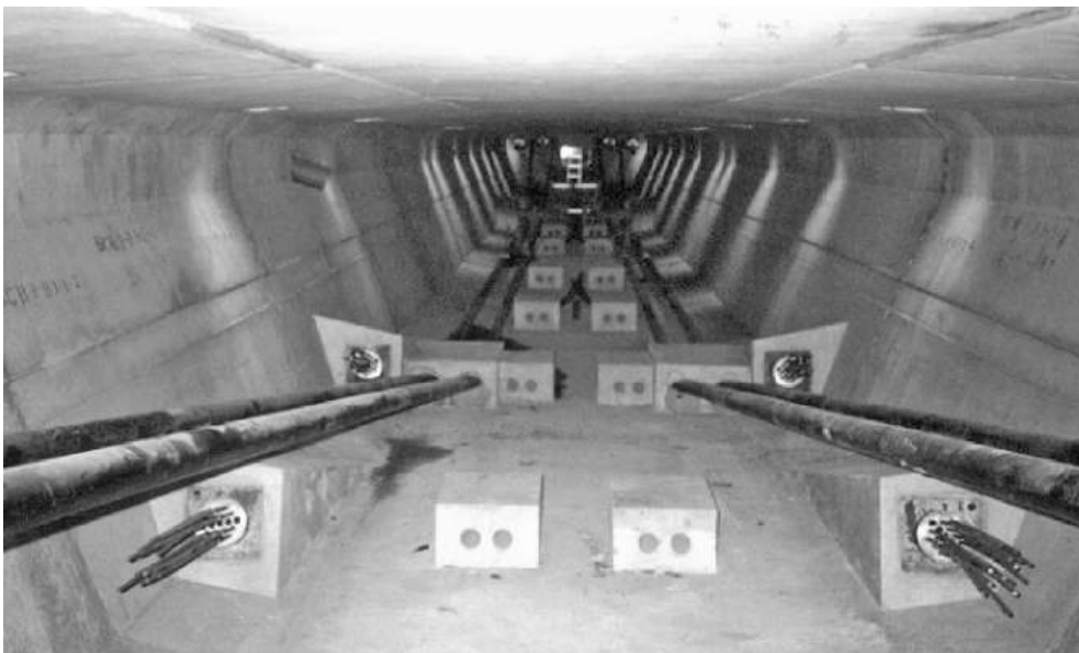
Figure 1.10 External tendons inside box girder deck
