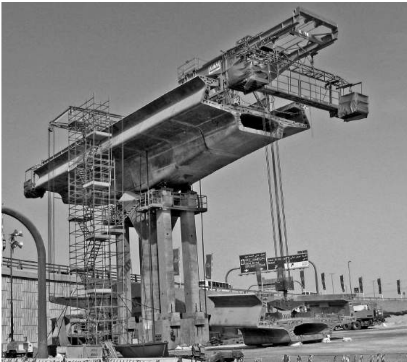
Figure 13.40 Precast segments erected by lifting frame
