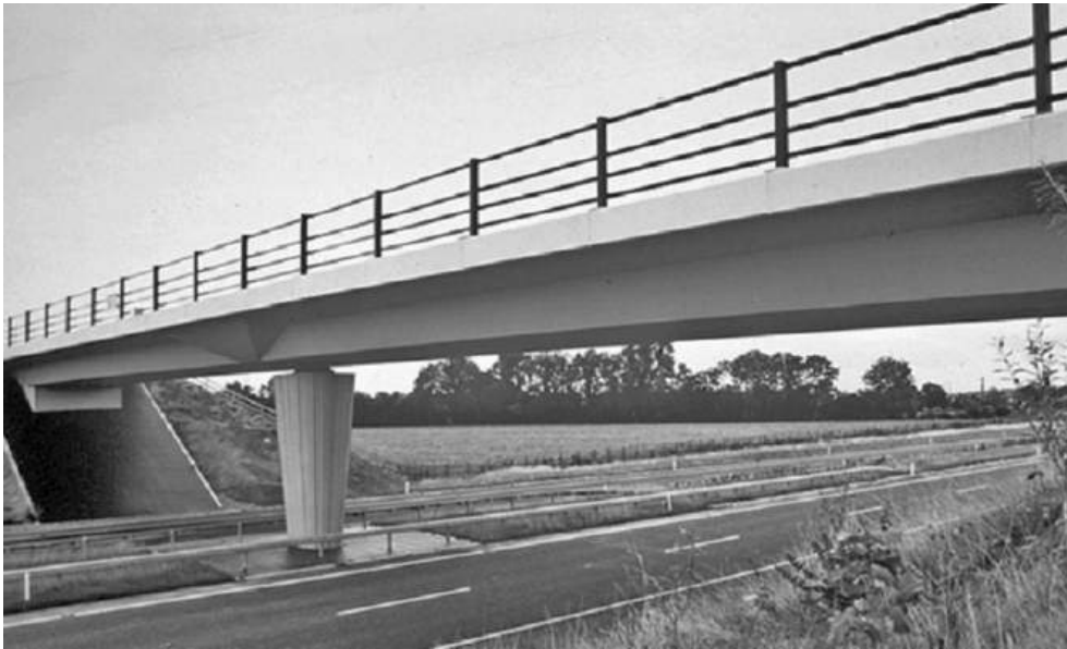
Figure 9.2 M4 Overbridge, Ireland (reproduced courtesy of Roughan & O'Donovan, Dublin, copyright reserved)
