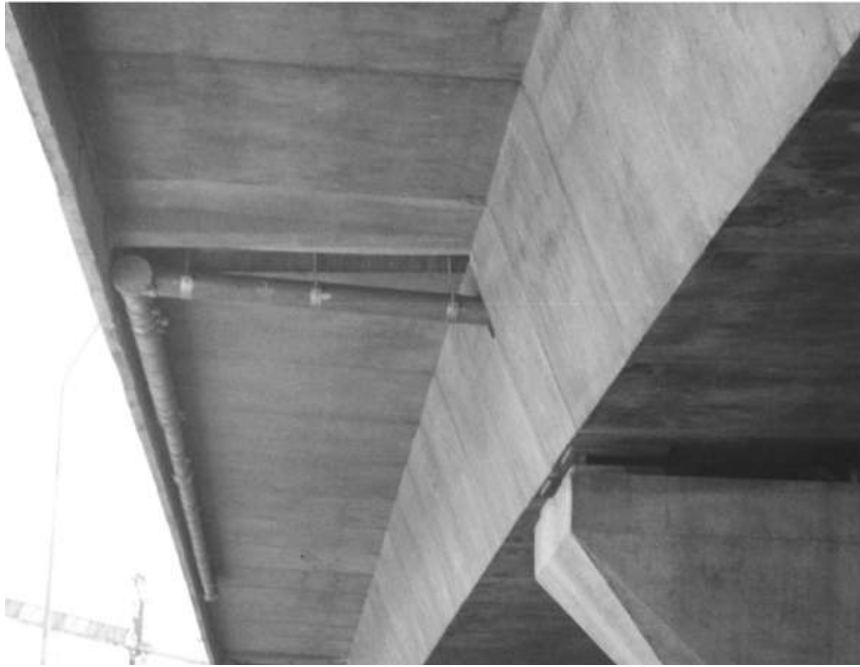
Figure 3.4 Deck drainage
