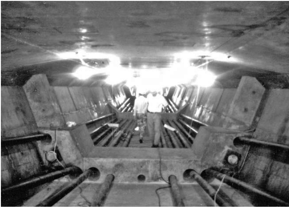
Figure 6.19 Concrete block deviator
