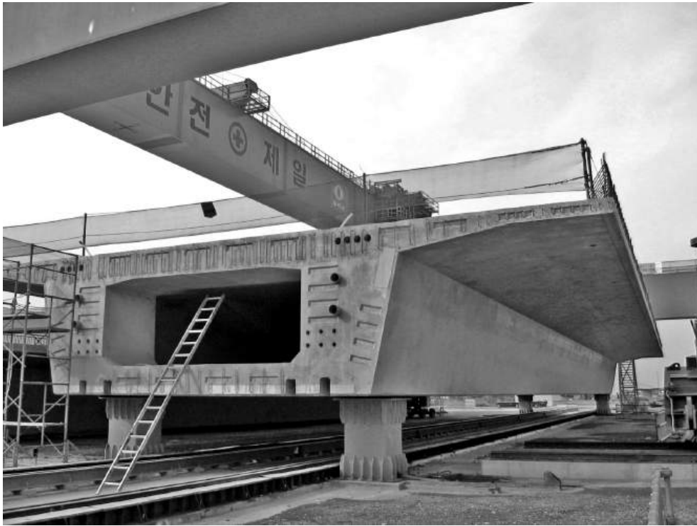
Figure 14.8 Completed precast unit stored
