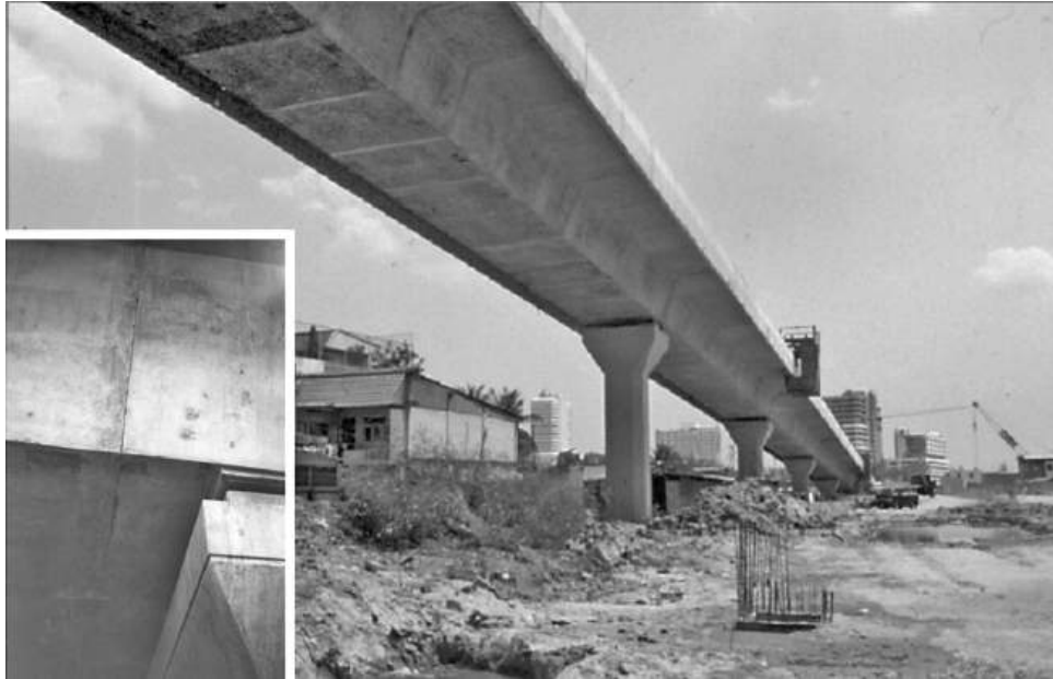
Figure 13.33 Dry-jointed segmental deck
