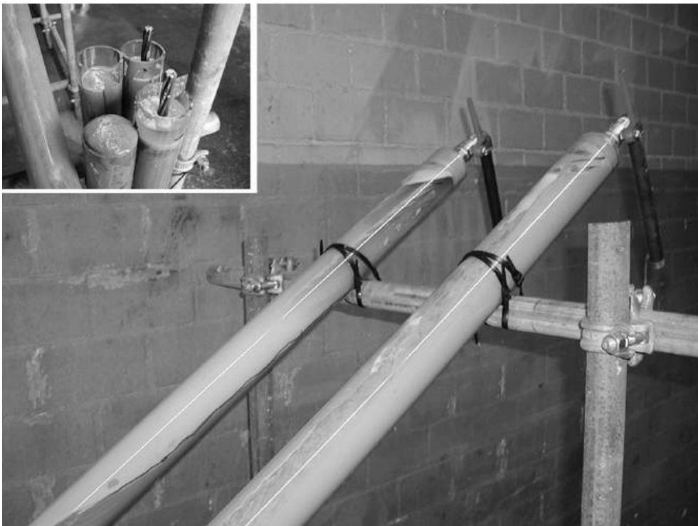
Figure 4.4 Inclined duct test (reproduced courtesy of VSL International, copyright reserved)
