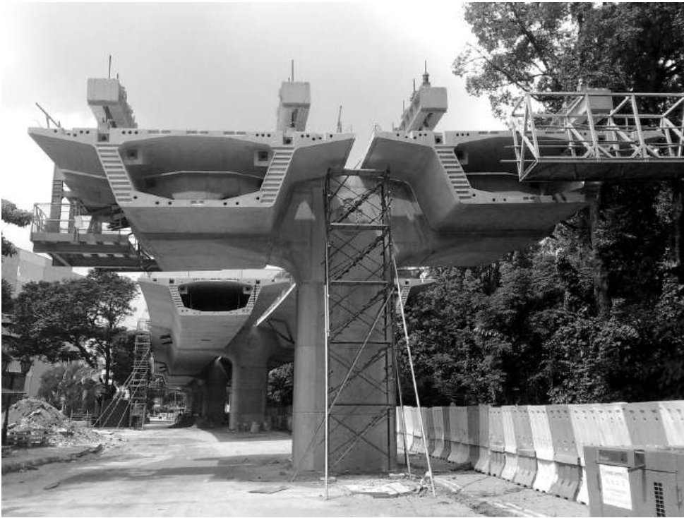
Figure 7.4 Precast segmental box girder (reproduced courtesy of H&T Associates, copyright reserved)
