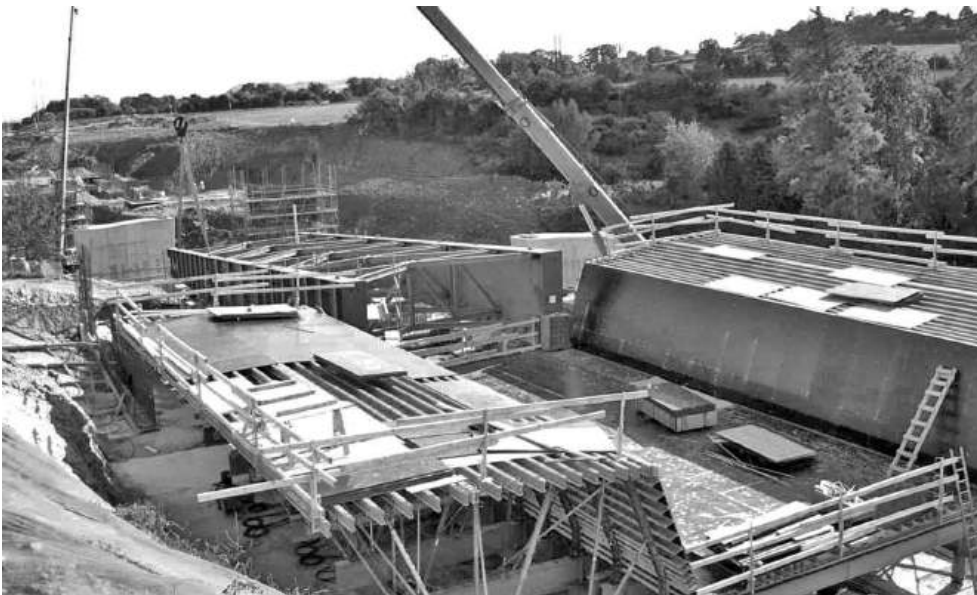
Figure 15.6 Casting bed behind abutment
