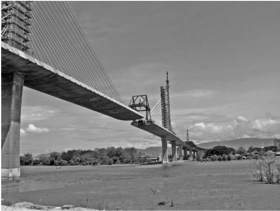
Figure 16.8 Lifting frame on deck for segment erection
