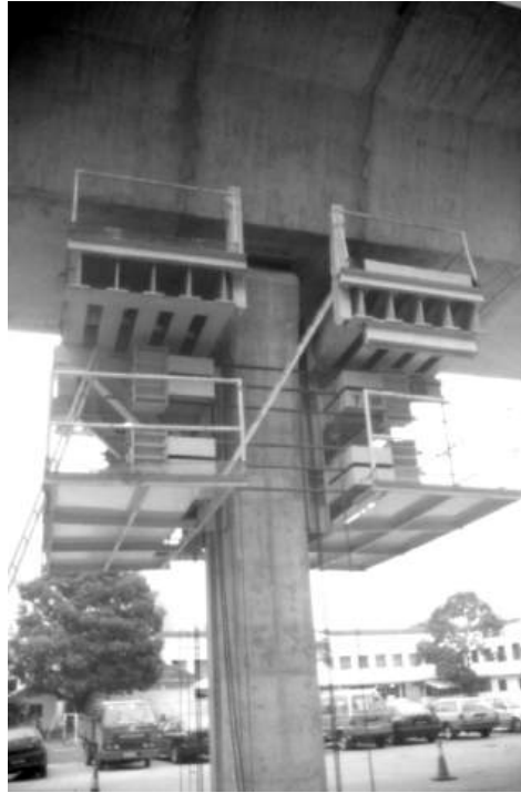
Figure 13.42 Deck cantilever supported off bracket fixed to pier
