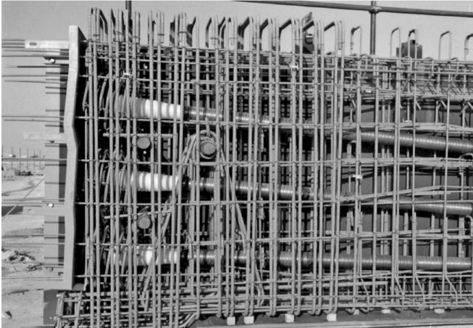
Figure 6.3 End block reinforcement with internal ducts
