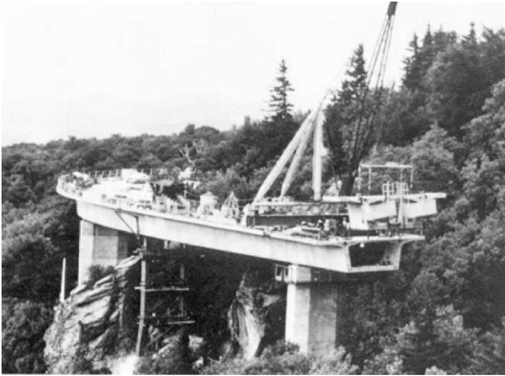
Figure 1.13 Linn Cove Viaduct, USA (reproduced courtesy of VSL International, copyright reserved)
