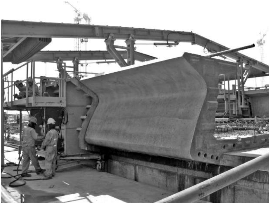
Figure 13.12 Segments on long line casting bed
