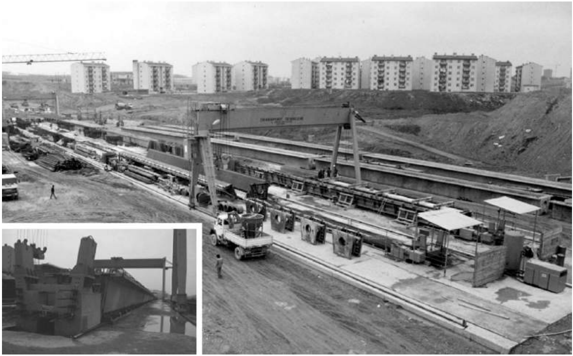
Figure 1.8 Precasting yard for the Bosphorus Crossing project, Turkey
