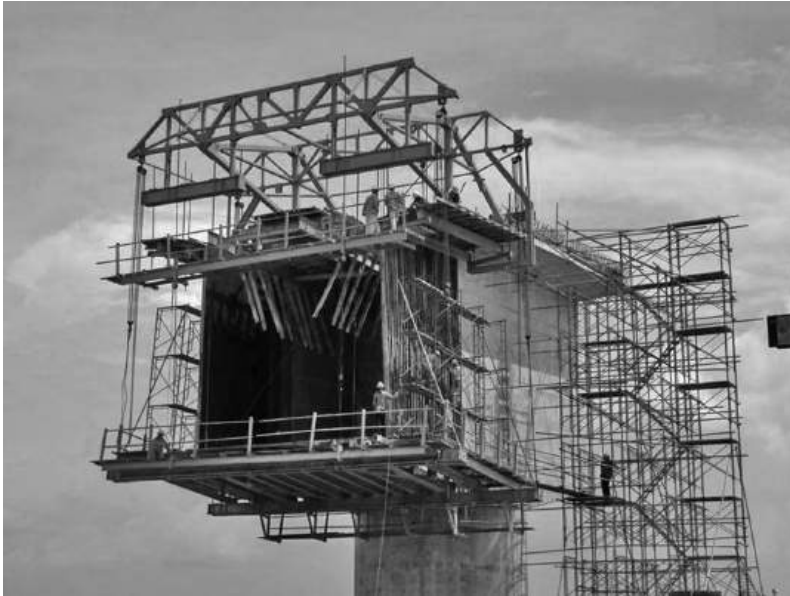
Figure 12.12 Pierhead and setting up traveller
