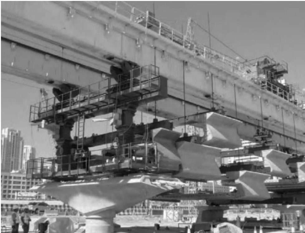
Figure D17 Freyssibar used in temporary works
