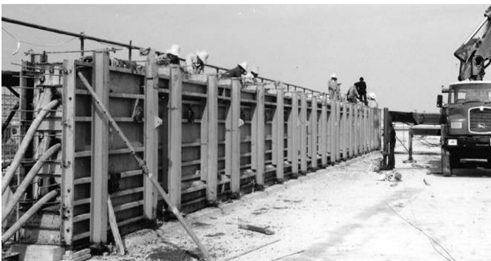
Figure 10.17 Shutter for post-tensioned precast beam (reproduced courtesy of Hyder Consulting (UK) Ltd, copyright reserved)
