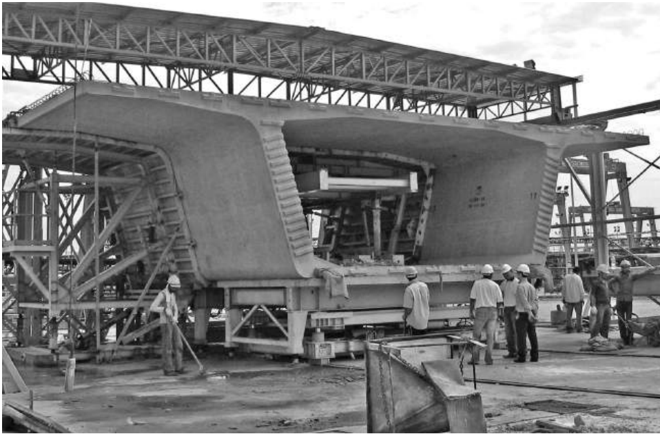
Figure 13.11 Counter-cast segment positioned
