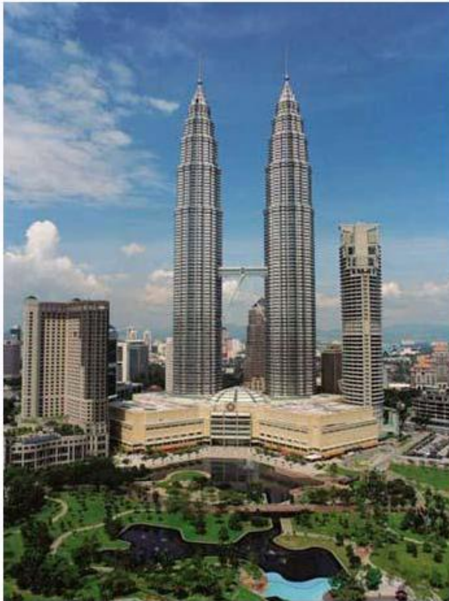
Figure1: PETRONAS twin tower
